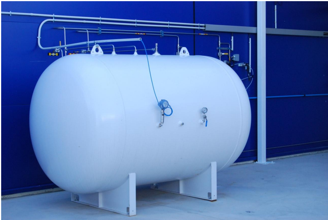
Illustration 3. Hydrogen Buffer
