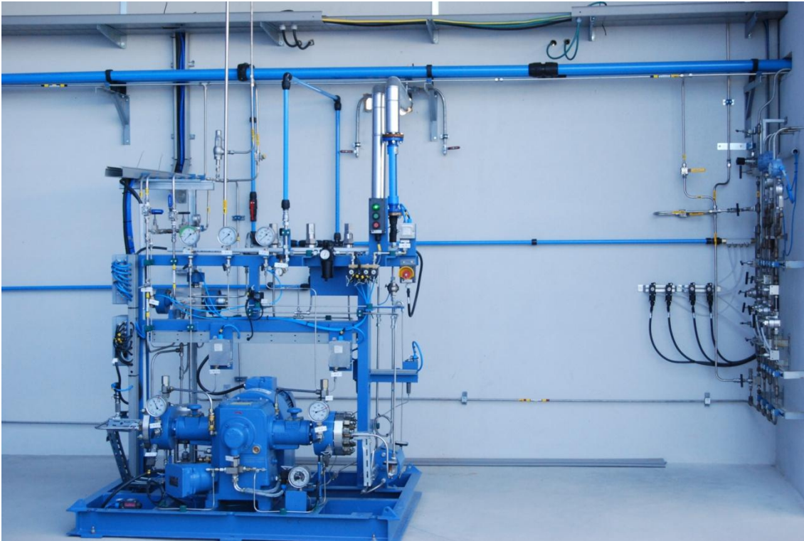
Illustration 4. Hydrogen compressor
