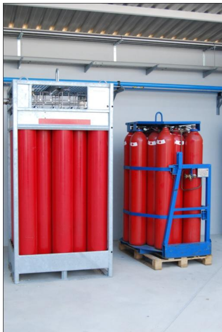
Illustration 5. Hydrogen storage system
