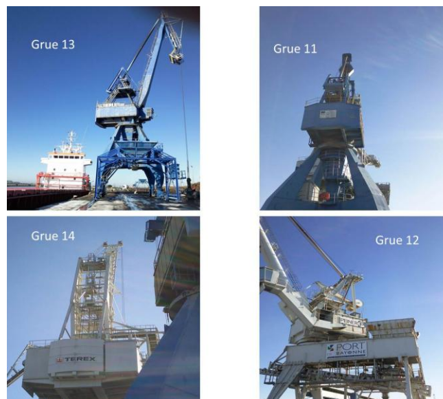
Illustration 7. Cranes on the wharf.
