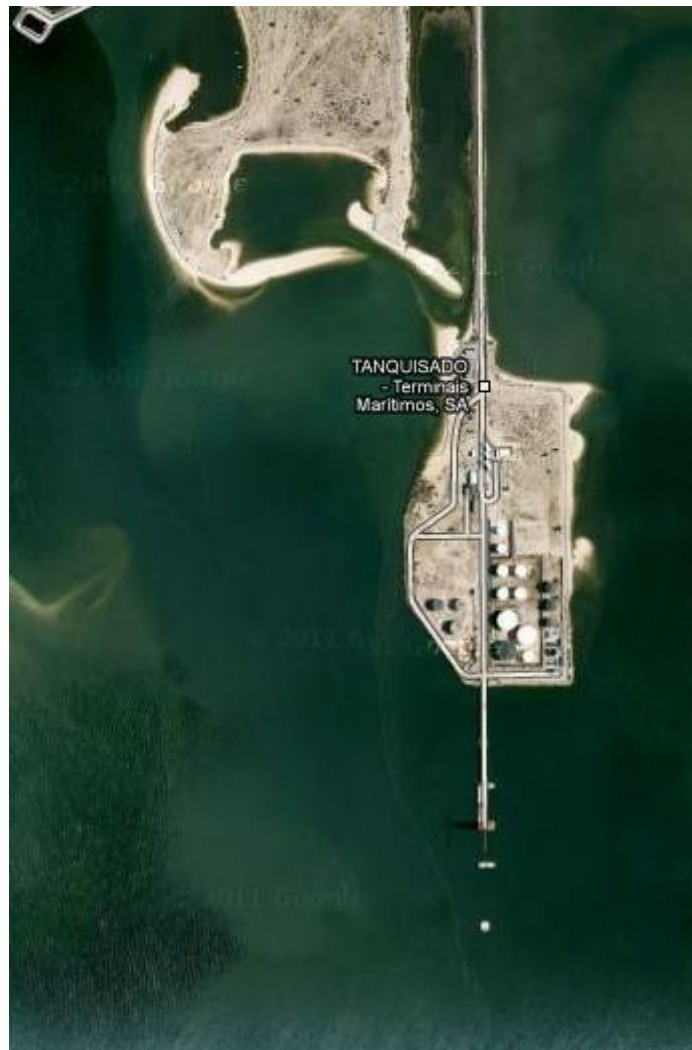
Fig. 5. Aerial view of the facility
