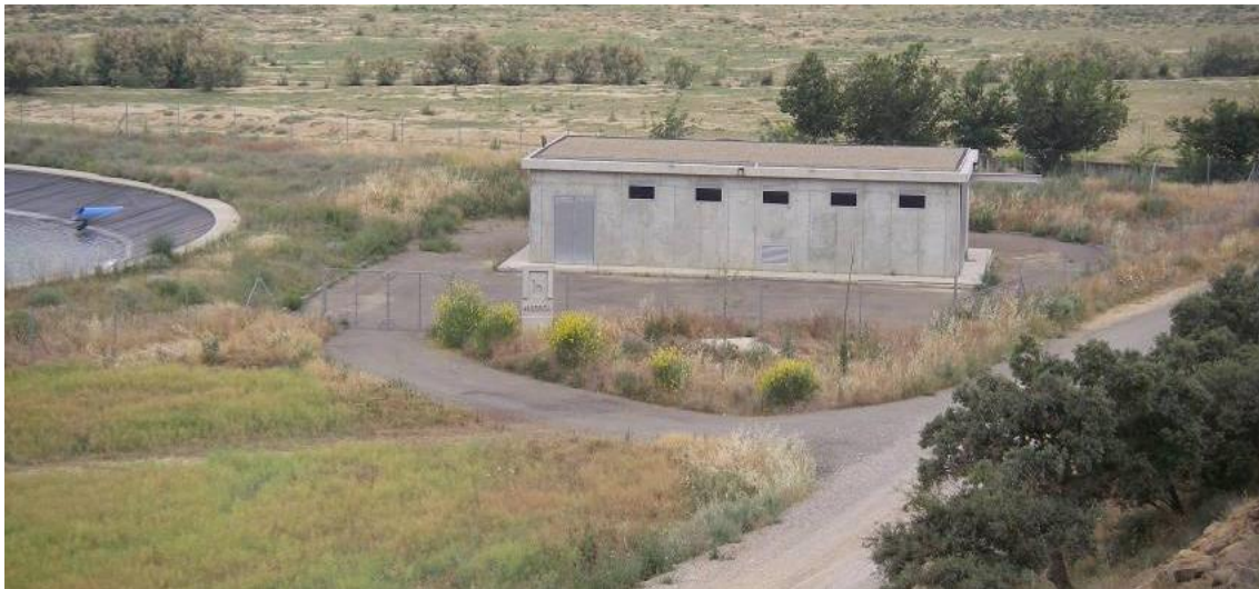
Ilustración 6. Building of the pumping station.
