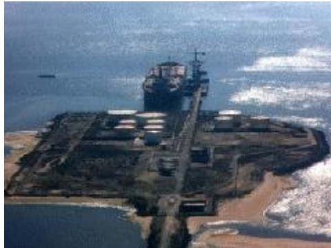
Fig. 4. Overview of the facility
